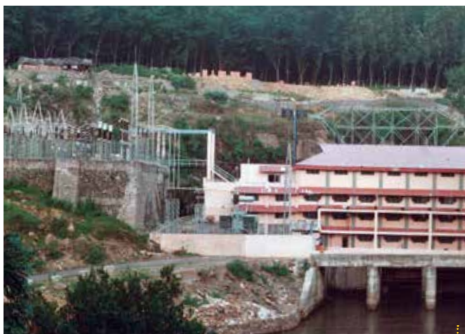
The Maniyar Hydroelectric plant, 1994
