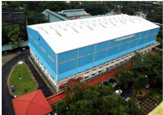
The silicon carbide micro grit plant at Kakkanad SEZ, 2009
