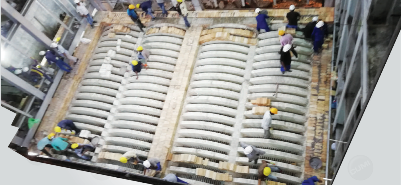
Rider Arch Construction at site
