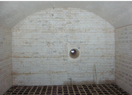
Fused Mullite Bricks for side wall, Target wall & Crown - CUMILITE WHF
