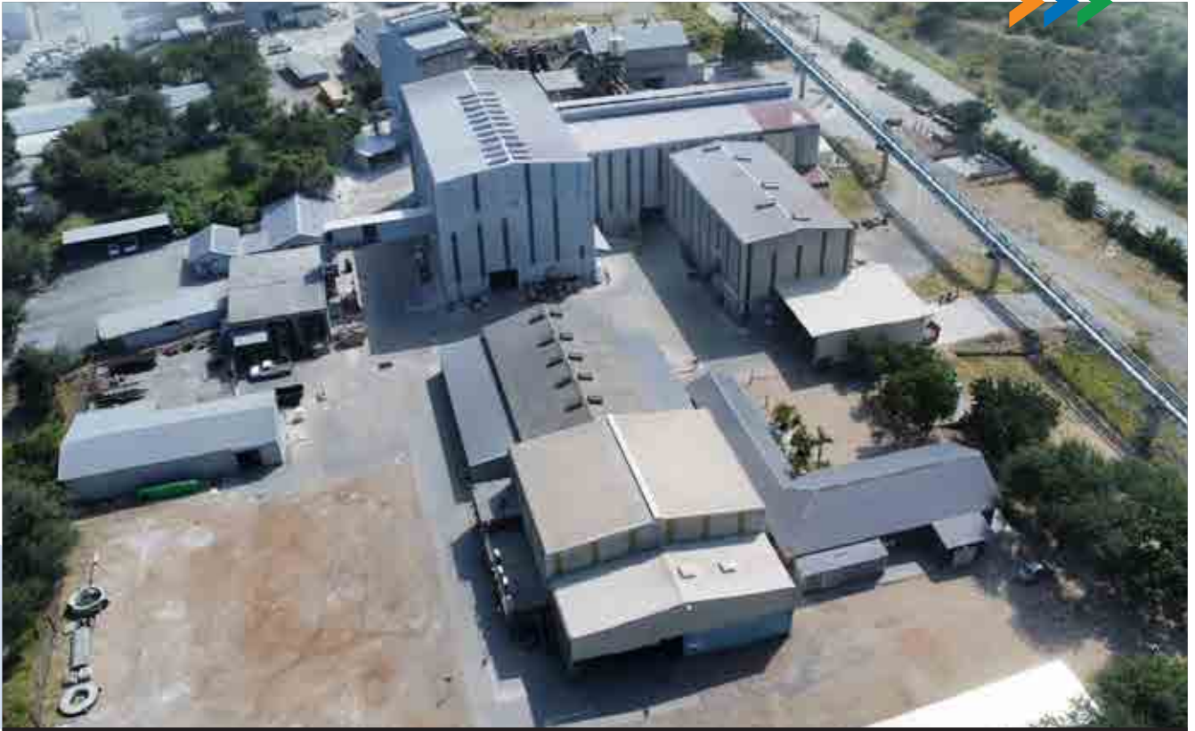
An aerial view of the Foskor Zirconia Plant at Phalaborwa, South Africa
