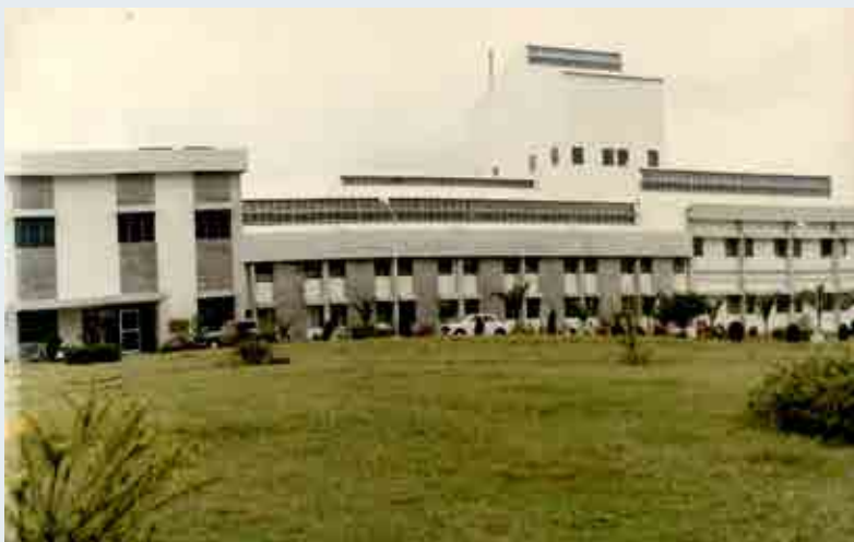
Industrial Ceramics plant in Hosur
